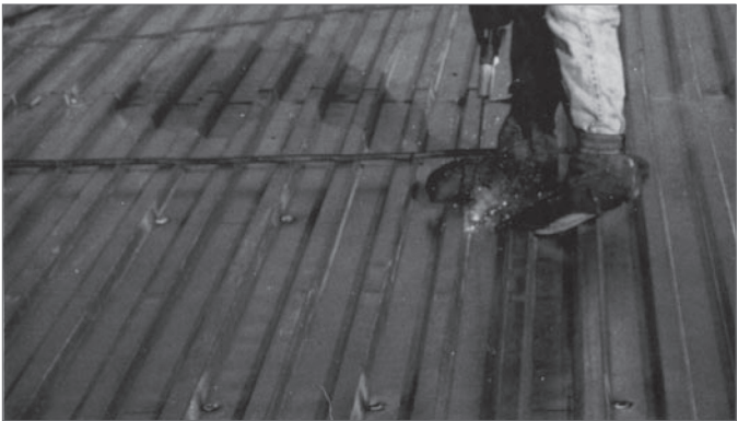
Fastening steel deck by welding.
